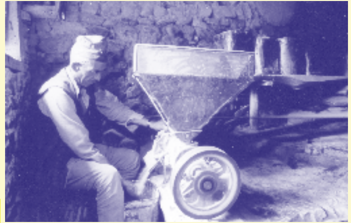
Paddy hullers attached to improved water mills are helping to reduce drudgery (Photo: CRT, Nepal)
